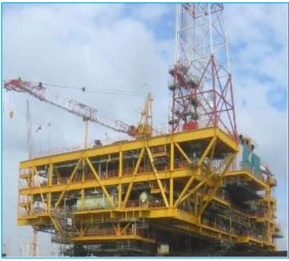
HELANG TOPSIDES PROJECT
