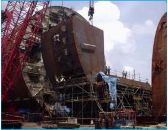
KIKEH DTU TRUSS SPAR PROJECT
