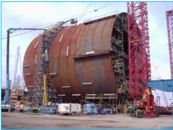
KIKEH DTU TRUSS SPAR PROJECT
