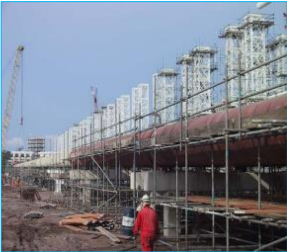
MLNG 3 SLUGCATCHER PROJECT
