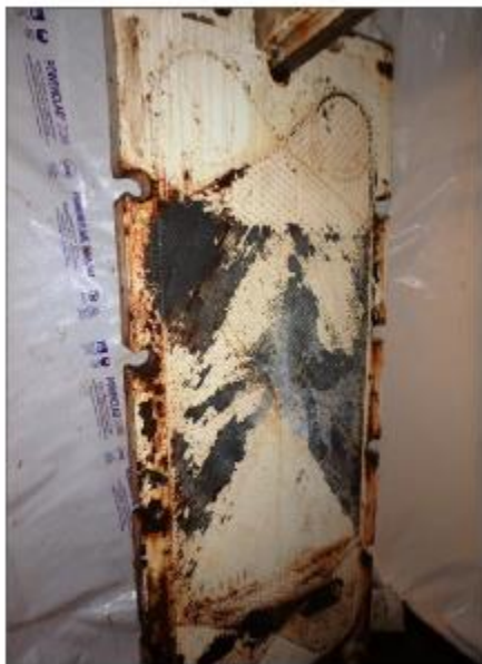
Backplate of cooler prior to repair
