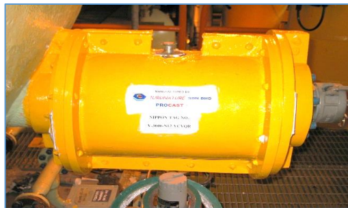
Valve casting sealed to the quick release connector's flange, to allow uninterrupted access to the quick release connector.
