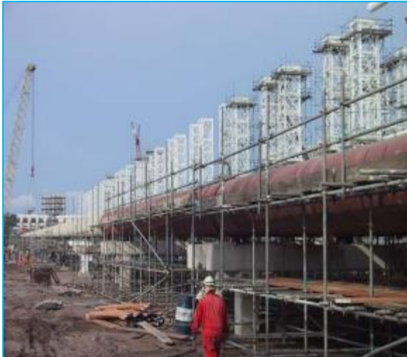
MLNG 3 SLUGCATCHER PROJECT
