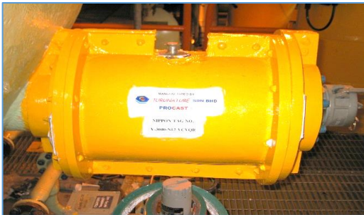
Valve casting sealed to the quick release connector's flange, to allow uninterrupted access to the quick release connector.
