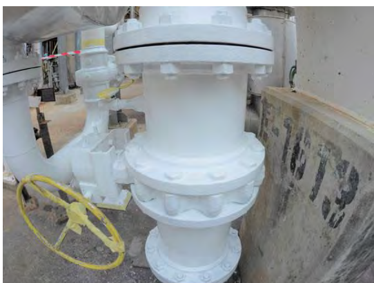
Coating applied during normal surface temperature
