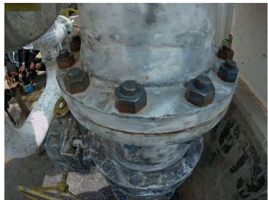
Mechanical preparation to ST2
