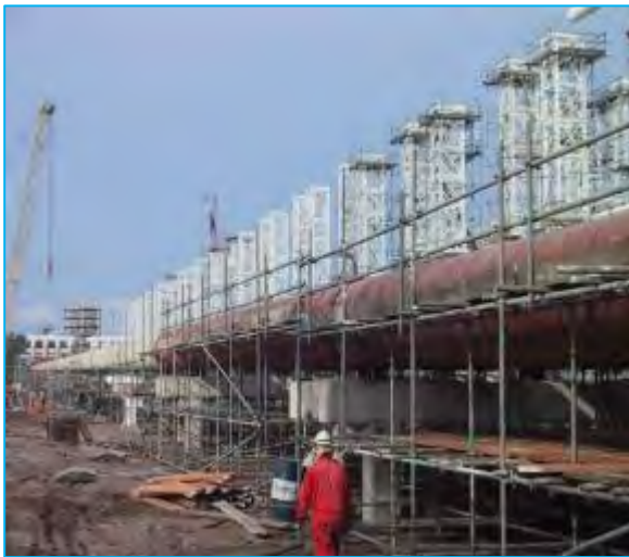
MLNG 3 SLUGCATCHER PROJECT
