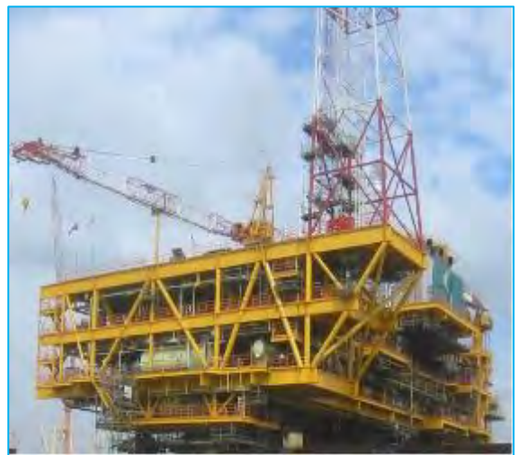
HELANG TOPSIDES PROJECT
