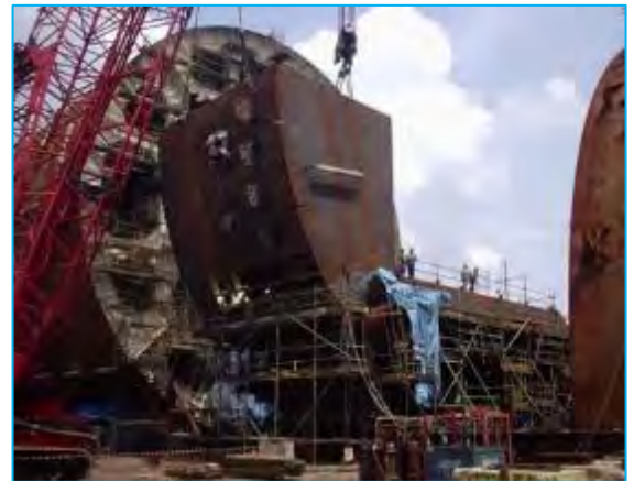
KIKEH DTU TRUSS SPAR PROJECT
