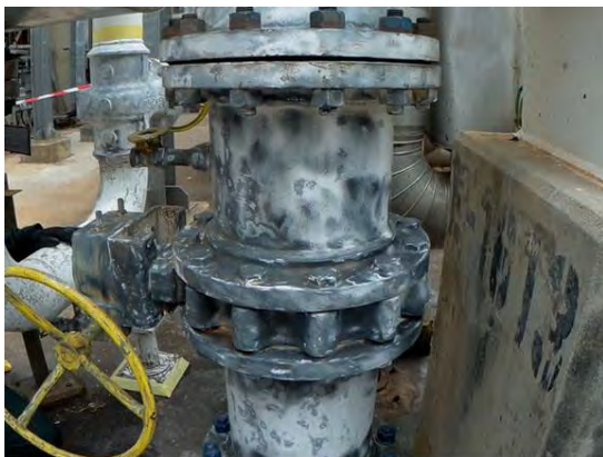
Mechanical preparation to ST2
