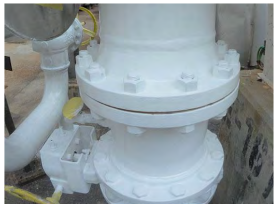
Coating applied during normal surface temperature
