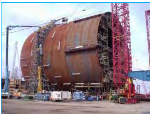
KIKEH DTU TRUSS SPAR PROJECT
