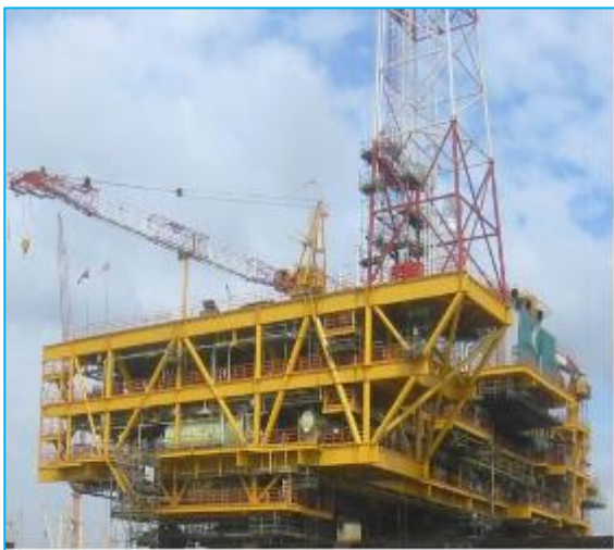
HELANG TOPSIDES PROJECT
