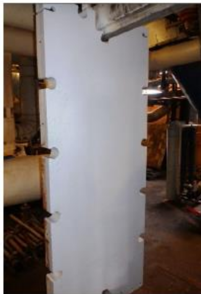
Coating repair with Humidur®
