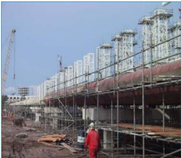
MLNG 3 SLUGCATCHER PROJECT
