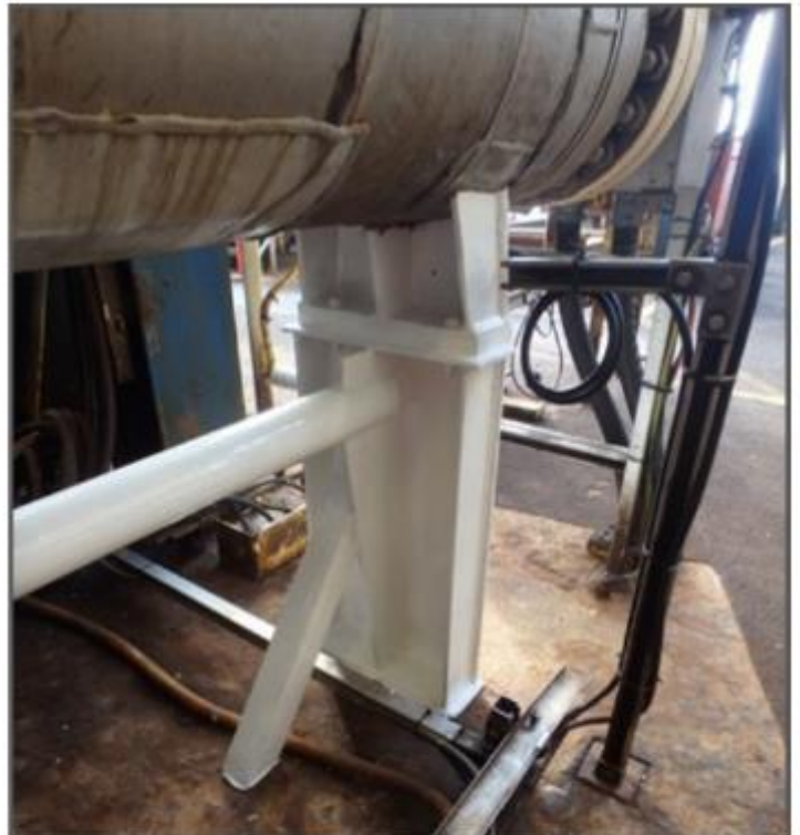
Support of vessel coated with Humidur®
