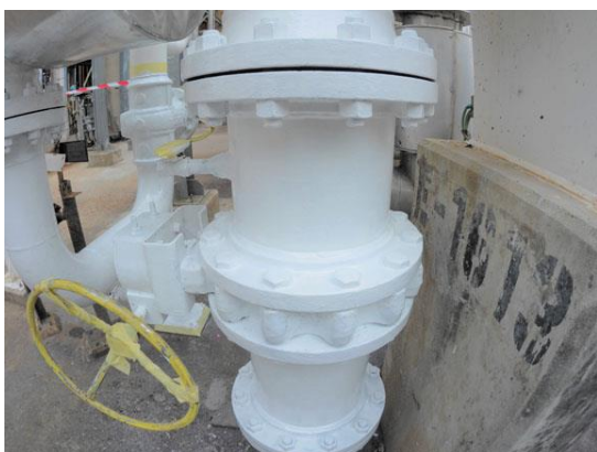
Coating applied during normal surface temperature
