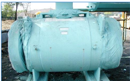
Valve body after wet application. Note, the nameplate and data plate have been left uncovered. They were later covered by removable PFP access panels.
