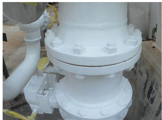
Coating applied during normal surface temperature
