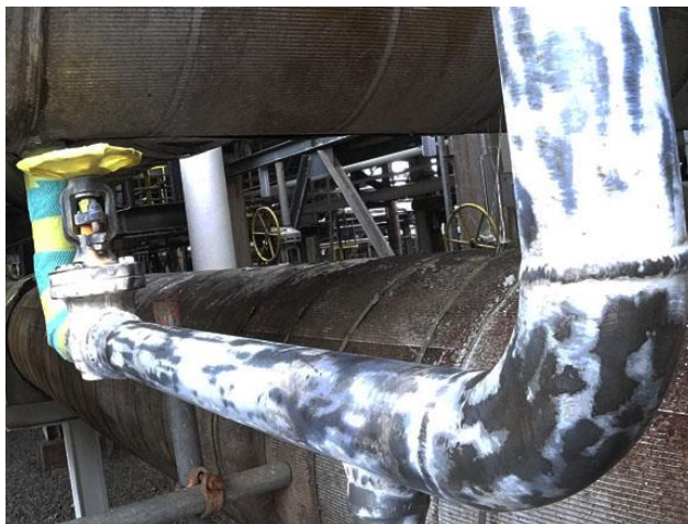
Mechanical preparation to ST2
