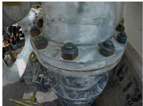
Mechanical preparation to ST2
