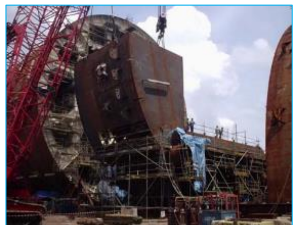
KIKEH DTU TRUSS SPAR PROJECT
