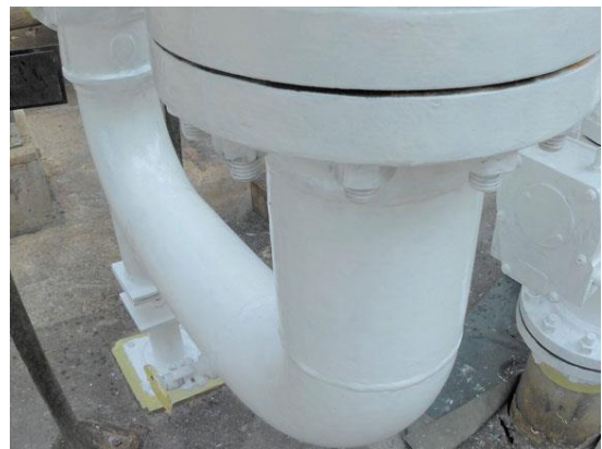
Coating applied during hot surface temperature
