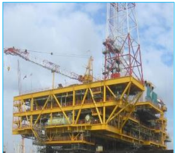
HELANG TOPSIDES PROJECT
