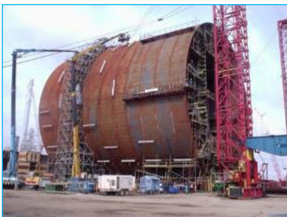
KIKEH DTU TRUSS SPAR PROJECT
