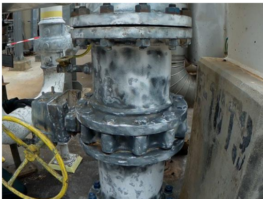
Mechanical preparation to ST2
