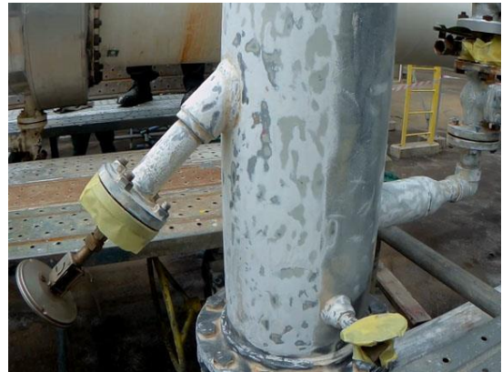
Mechanical preparation to ST2
