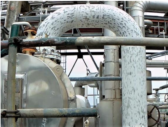
Mechanical preparation to ST2
