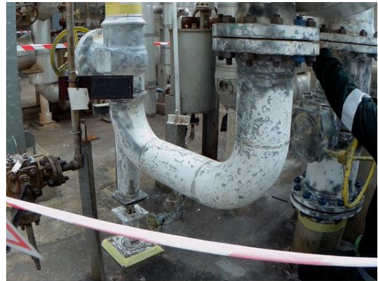
Mechanical preparation to ST2
