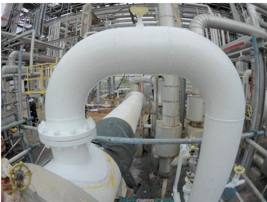
Coating applied during hot surface temperature
