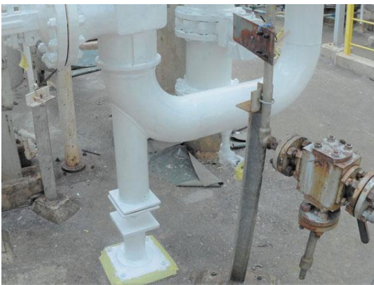
Coating applied during hot surface temperature
