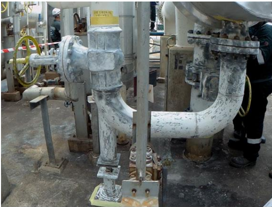
Mechanical preparation to ST2
