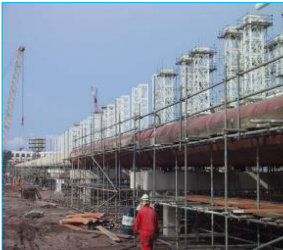
MLNG 3 SLUGCATCHER PROJECT
