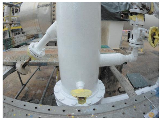
Coating applied during hot surface temperature
