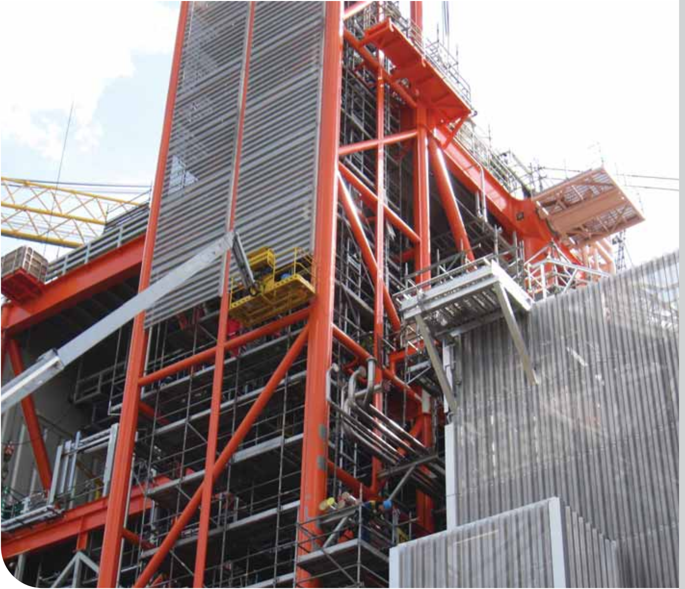
BP Valhall stair tower heatshields and deck wind wall systems
