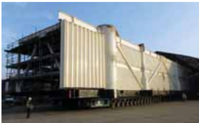
Apache Forties Alpha fire and blast walls
