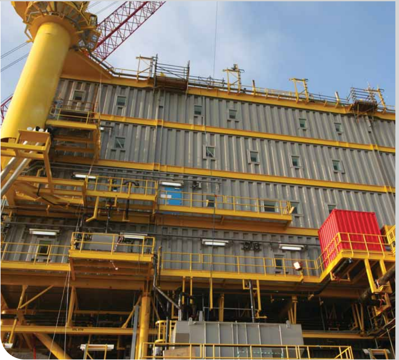
Maersk Al Shaheen LO, fire and blast wall installation
