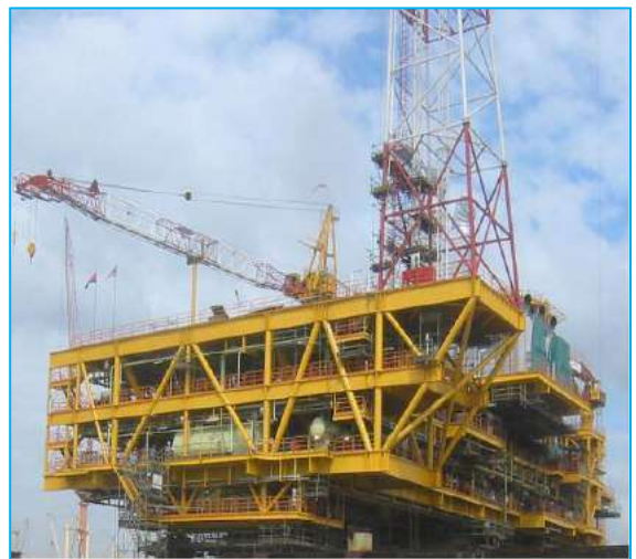
HELANG TOPSIDES PROJECT
