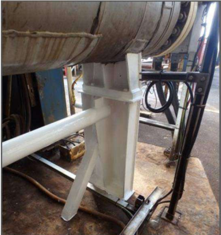
Support of vessel coated with Humidur®
