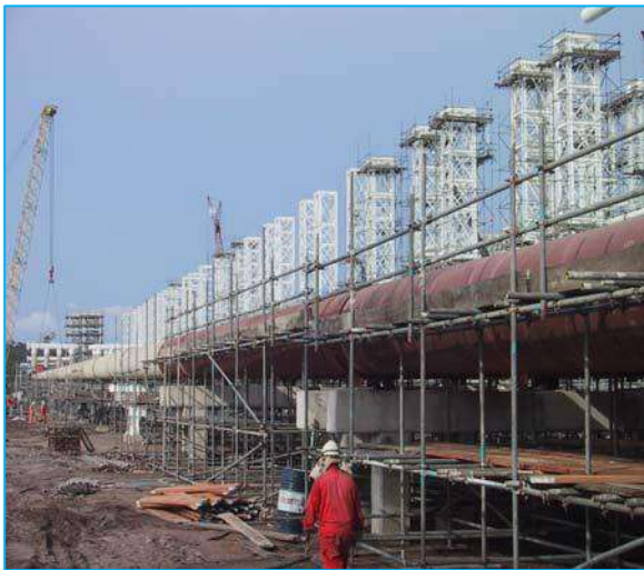
MLNG 3 SLUGCATCHER PROJECT
