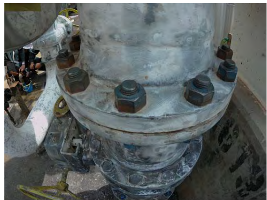
Mechanical preparation to ST2
