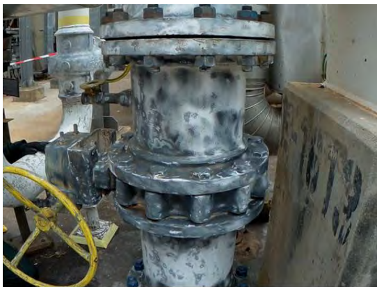
Mechanical preparation to ST2
