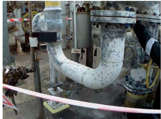
Mechanical preparation to ST2
