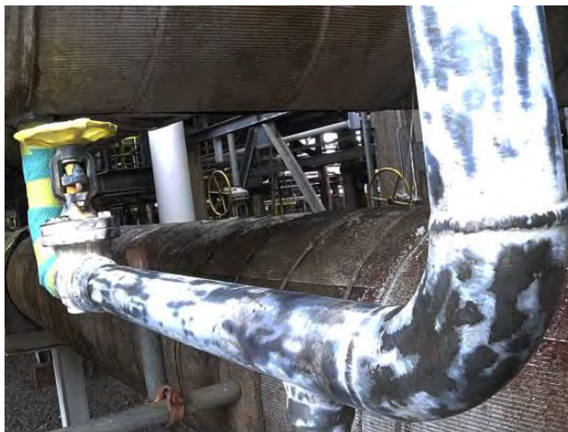
Mechanical preparation to ST2
