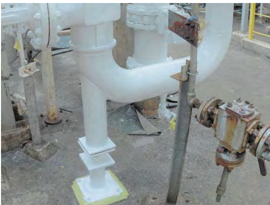
Coating applied during hot surface temperature
