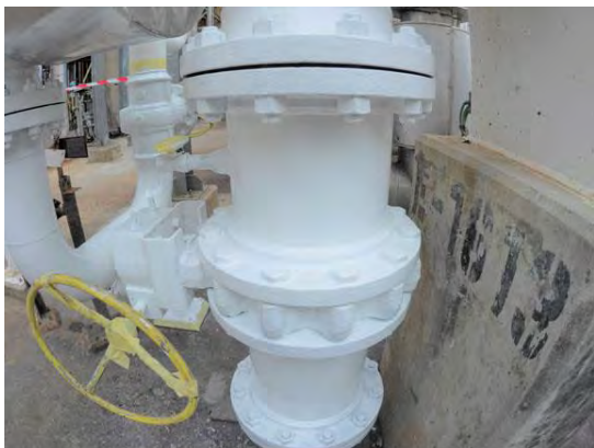
Coating applied during normal surface temperature
