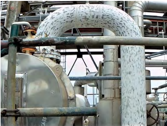
Mechanical preparation to ST2
