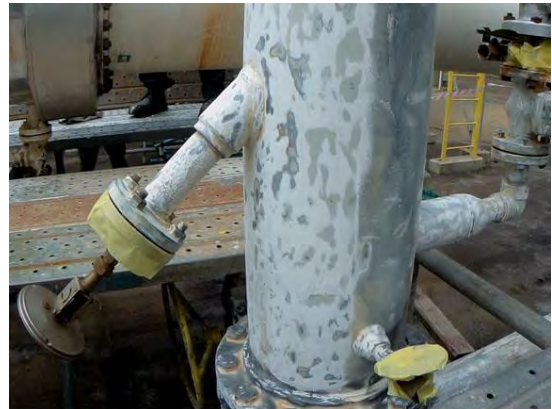
Mechanical preparation to ST2
