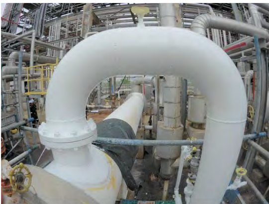
Coating applied during hot surface temperature
