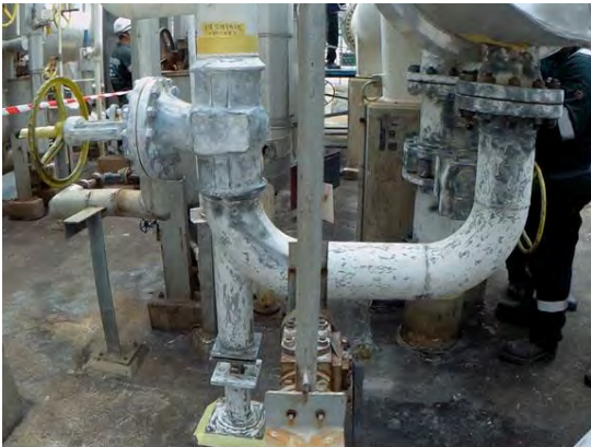
Mechanical preparation to ST2
