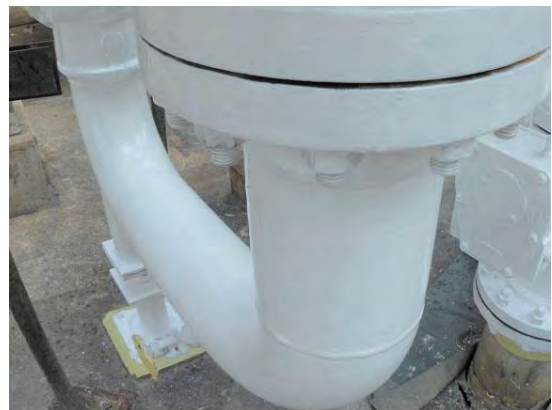
Coating applied during hot surface temperature
