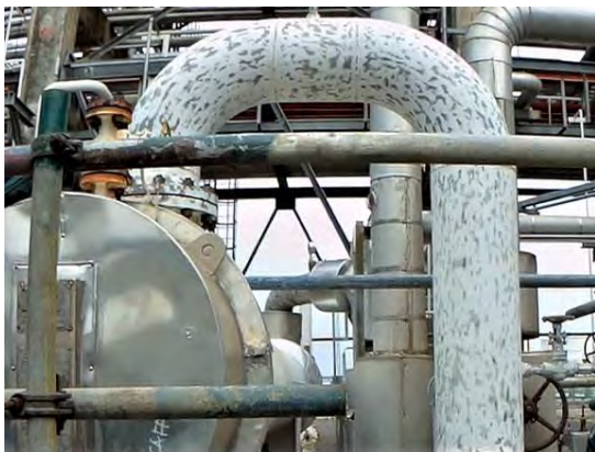
Mechanical preparation to ST2
