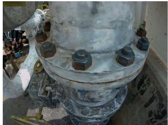
Mechanical preparation to ST2
