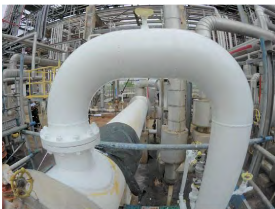
Coating applied during hot surface temperature
