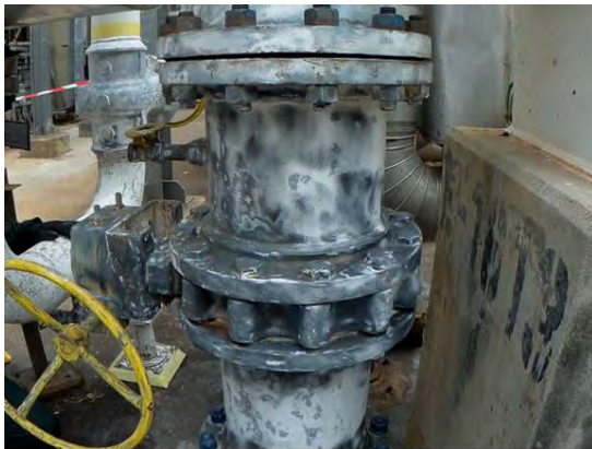
Mechanical preparation to ST2
