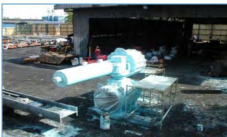
SDV after wet application and all but the flange castings are completed. The flange covers were to be fitted offshore, after installation of the valve.
