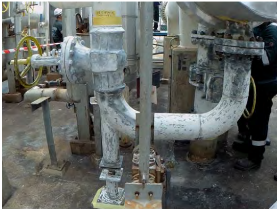
Mechanical preparation to ST2
