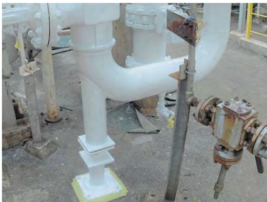
Coating applied during hot surface temperature
