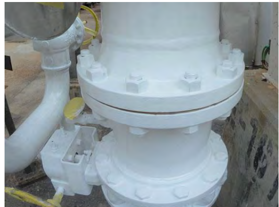
Coating applied during normal surface temperature
