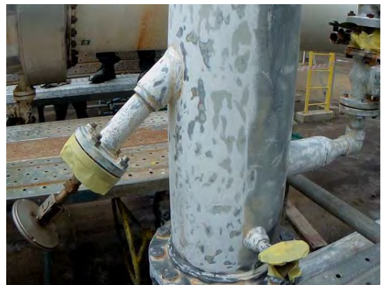
Mechanical preparation to ST2
