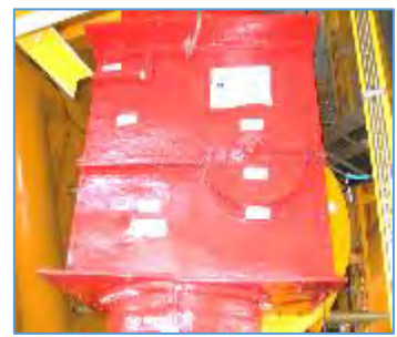
Completed 36" Main SDV, installed and fitted with its PFP castings and wet applied PFP .
