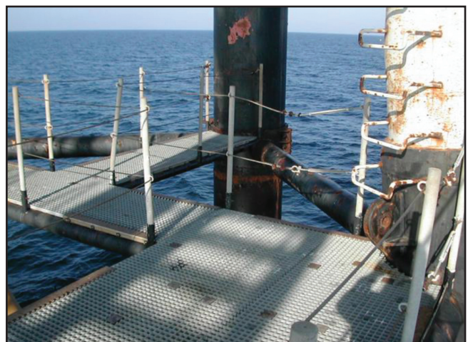
AIMS Fiberglass Grating System after 16 years of service
